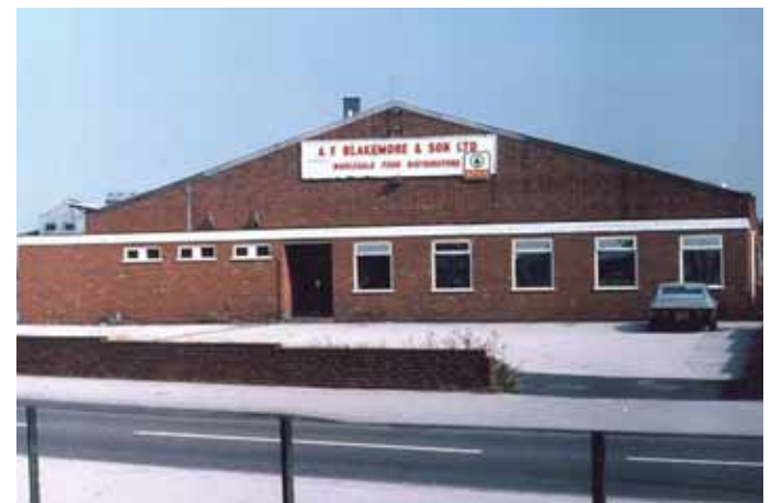
A.F. Blakemore's former cash & carry and delivered warehouse, located at Leamore Lane, Walsall
